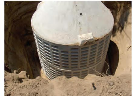
Typical precast concrete drywell
