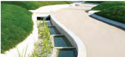
Tiered rainwater channel on slope
