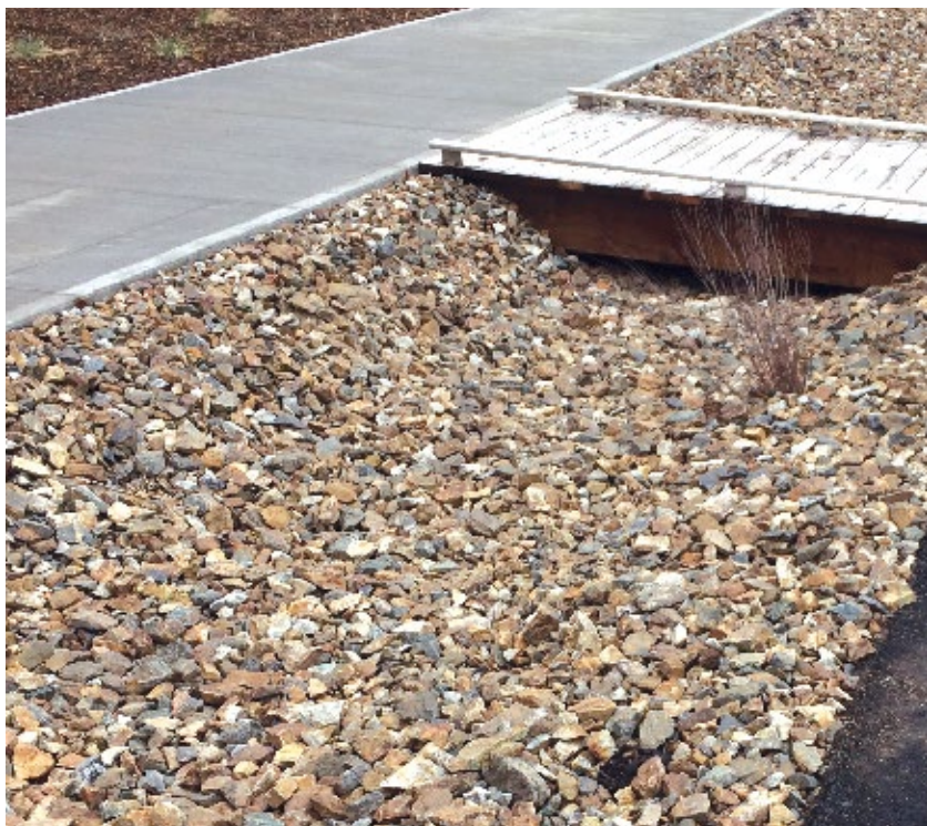
Bioswales into the Mountain Weather Office parking lot
